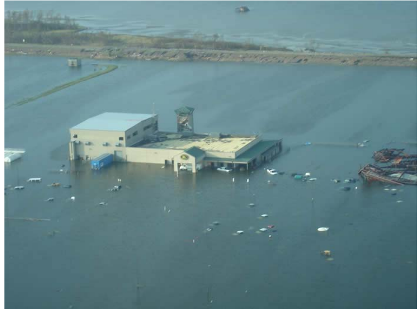
Petroleum Helicopter Inc. – Boothville
