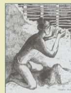
Applying daub (clay with Spanish moss) to wattle to create a wall.
